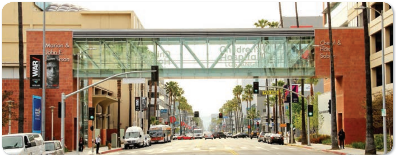
The new bridge over Sunset Boulevard connects wings of the CHLA campus
